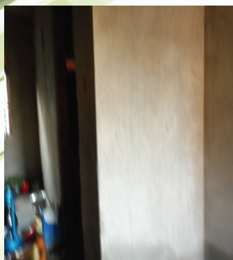
Plastered walls inside all bedrooms to reduce on dust.
