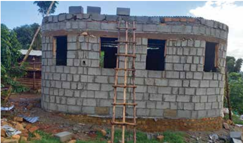
Sanitation facilities being constructed at Angel's Centre.
